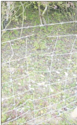
■ Damage to fences in Bredhurst
